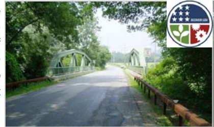
Lime Kiln Road Bridge in Dover
