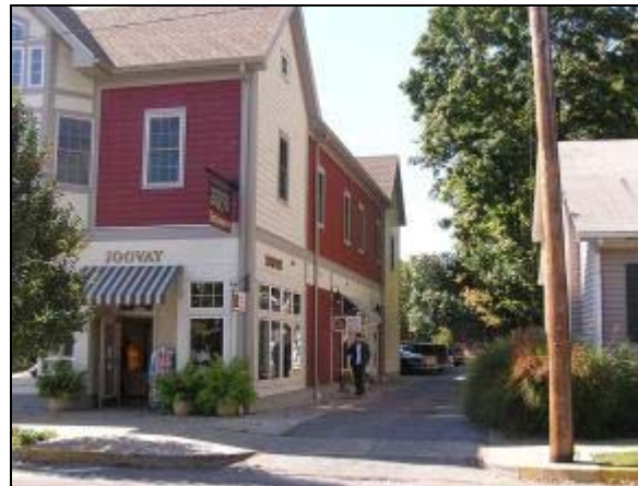
#4: This new one-way connection to Garden Street has helped make businesses in that previously dead-end area of the Village Center more successful.
