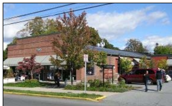
#2: A former auto dealership and garage was transformed into attractive shops, a bookstore, and a restaurant with patio seating out front.
