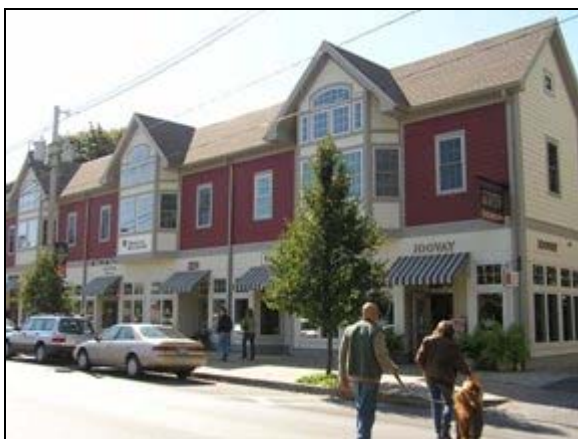
#1: A two-story 28,000 square foot retail/office building, winner of a 2005 Dutchess County Planning Federation award, replaced a vacant car sales lot.
