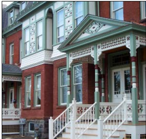
This development in Poughkeepsie involved the historic restoration of seven Queen-Anne style townhouses into seven affordable two-family homes.
