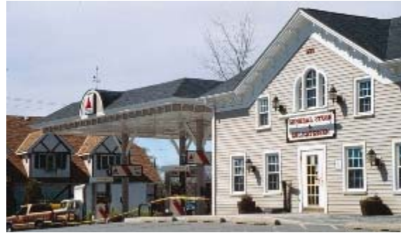
This side canopy in LaGrange was designed to reflect the roofline and cornice details of the old store building.
