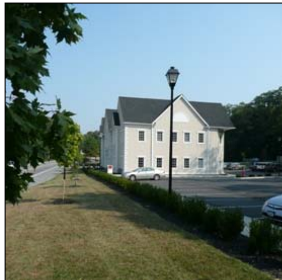
The redesigned Glenham Professional Plaza in Fishkill shows parking to the side and rear, improved landscaping, and minimal grading.
