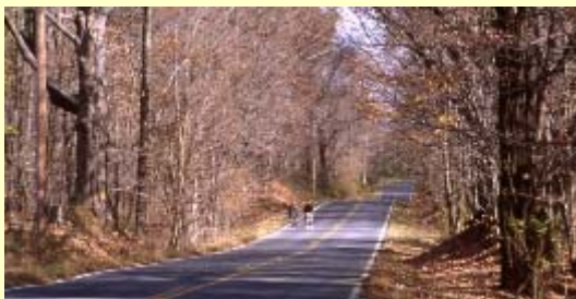
Wide vegetation clear zones are unnecessary on lower volume rural roads - 10 feet is desirable for all-purpose rural roads or at curves, and 2 to 5 feet for low-volume access roads under 40 mph. 1
