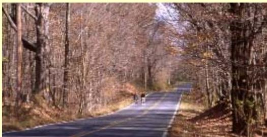
*Wide vegetation clear zones are unnecessary on lower volume rural roads - 10 feet is desirable for all-purpose rural roads or at curves, and 2 to 5 feet for low-volume access roads under 40 mph.<sup>1</sup>*
