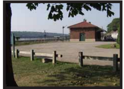
The parking lot at the Hyde Park Train Station will be improved using CDBG money for paving, curbs, drainage, landscaping and historic lighting. It will provide a safe parking area for residents to visit the former railroad station, use the Town Park and enjoy the beauty of the Hudson River.
