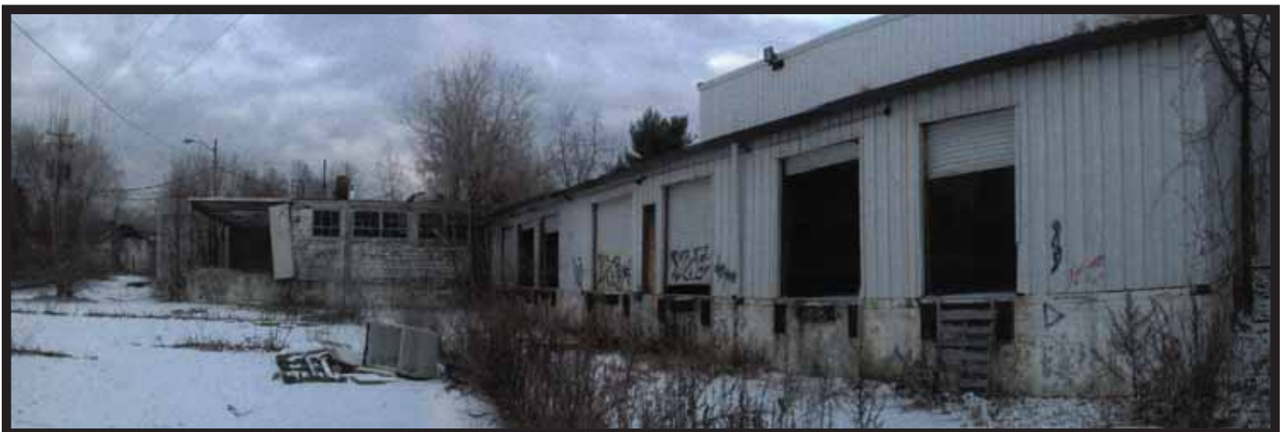
Some of the buildings to be demolished as part of the environmental restoration phase of the Perx project.
