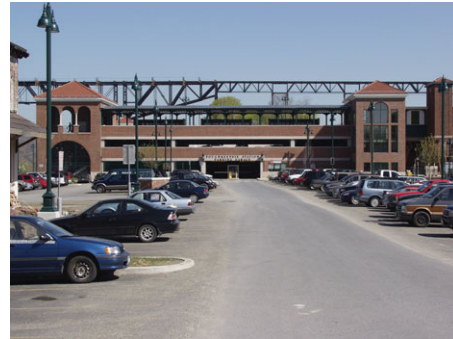
Metro-North expanded and improved parking with construction of a new parking deck at Poughkeepsie.
